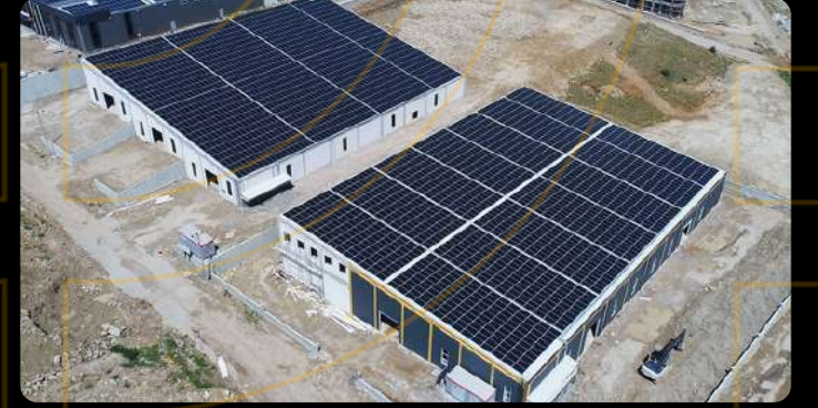
KONYA - BEYŞEHİR OSB GES - 1255KWP
