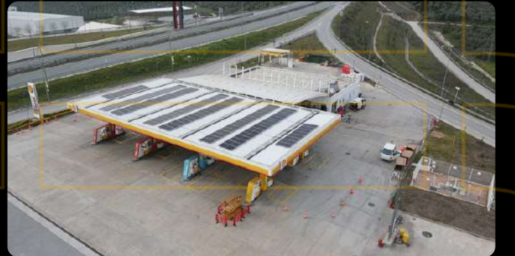
İZMİR/İSTANBUL - SHELL GES - 50KWP
